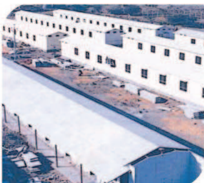
Reliance Petroleum Ltd. (Staff Accommodation) Mothikhavadi, Jamnagar, Gujarat
